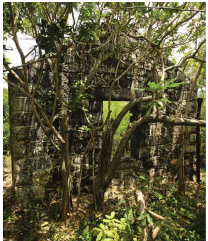
Vestiges of the Quarantine Station on Flat Island (Source: AGTF Collection)
