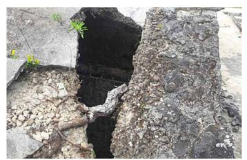
Part of the roof of chamber 8 had collapsed due to proliferation of roots
