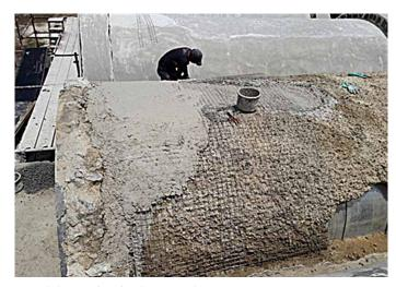
Consolidation of roof with wire mesh
