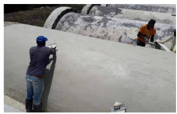
Laying of fresh lime mortar
