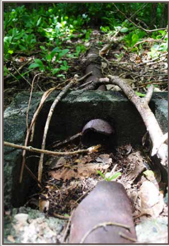
Water system at Flat Island.
